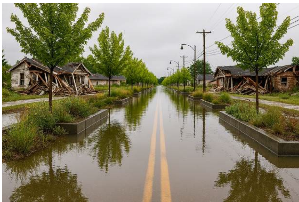
Figure 5. Flooded street with damaged houses, swales, and boxed trees. Author image.
