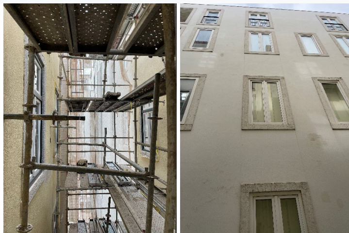
Figure 5. View of the rear façade renovation works
