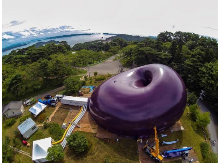
Figure 6. Aerial view of the Ark Nova transportable performance venue. 13
