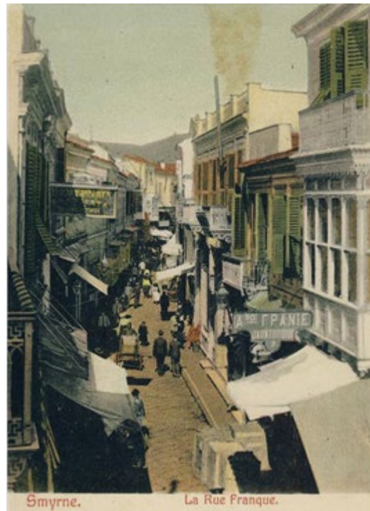
Figure 6. A view from the Frank Street. Source: Levantine Heritage .
