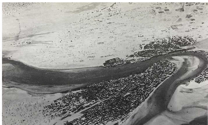
Figure 1. Image showing the Dubai Creek and organic developments
