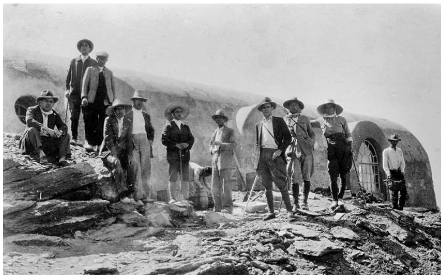
Figure 5. Construction of Elorrieta shelter between 1931-1933.
