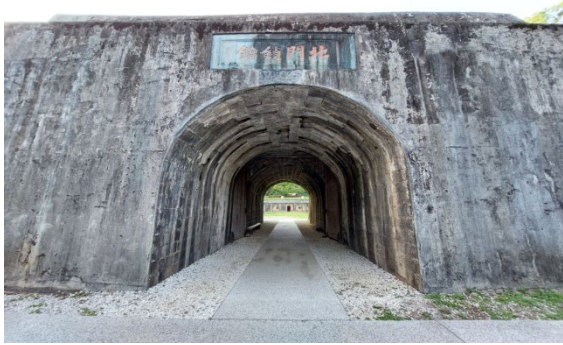
Figure 2. Entrance of Hobe Fort (image source: Author)
