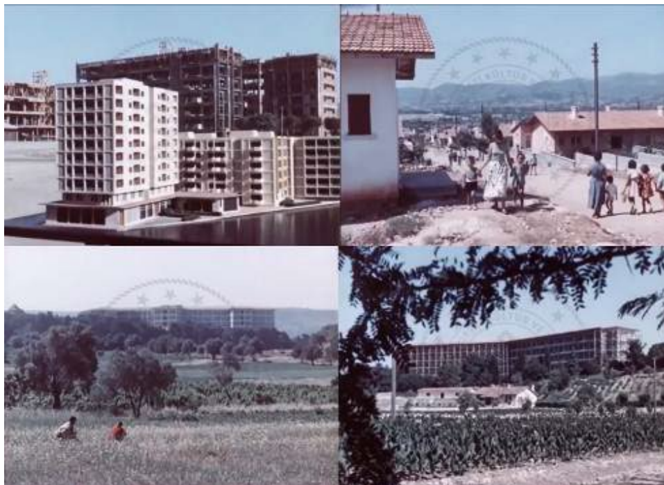
Figure 3. Upper row: The architectural model and the construction site of a new housing facility in Izmir. Lower row: Buca Sanatorium in Izmir. Source: “Let’s Get to Know Our Country: Izmir” (1955).
