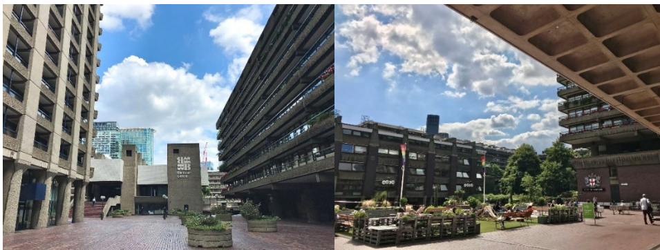
Figure 1. Entrance and the inner courtyard of the Barbican Centre
