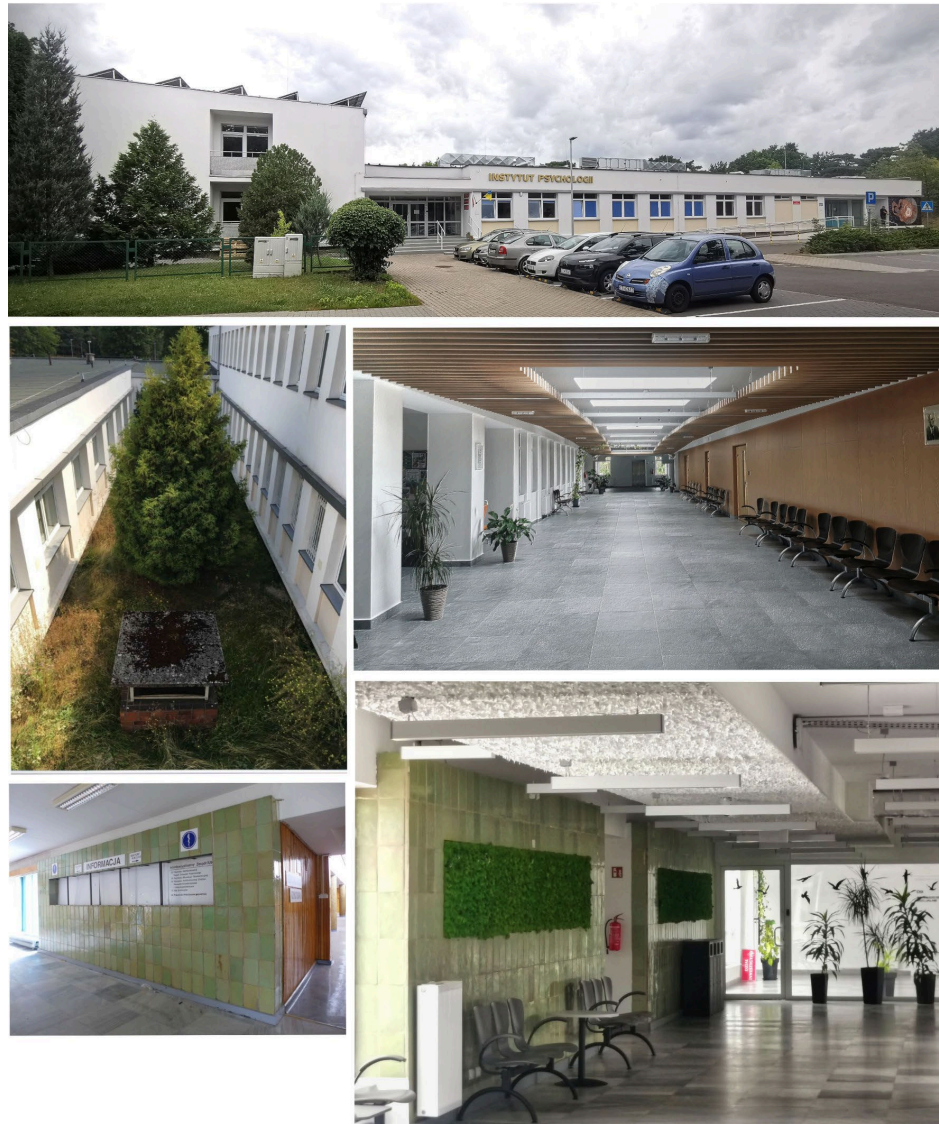
Figure 7. Toruń, NCU: the Institute of Psychology (photo. K. Zimna-Kawecka, 2024). Left: south patio and interior of east corridor with ceramic tile cladding and wainscoting before renovation (photo. M. Trojan. Chronicle of Headquarters construction of the Institute of Psychology NCU, July 2019, http://psychologia.umk.pl/Infokat/kronika-budowy/kronika-budowy-lipiec-2019 accessed August 28, 2024). Right: the new south corridor in place of the patio and east corridor with preserved former interior elements (photo. K. Zimna-Kawecka, 2024).
