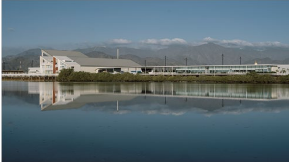
Figure 7. The Kalba Ice Factory, image provided by 51-1 Arquitectos
