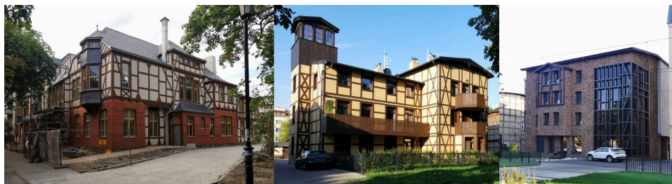
Figure 5 Toruń, three timber-frame buildings in Bydgoskie District, from left: historical monument subjected to conservation and restoration works (real authenticity); reconstructed/rebuilt monument (authenticity of form), contemporary building in place of the previous one with reference to the timber-frame construction (with reference to the genius loci of the place) (photo. Karolina Zimna-Kawecka, 2023)
