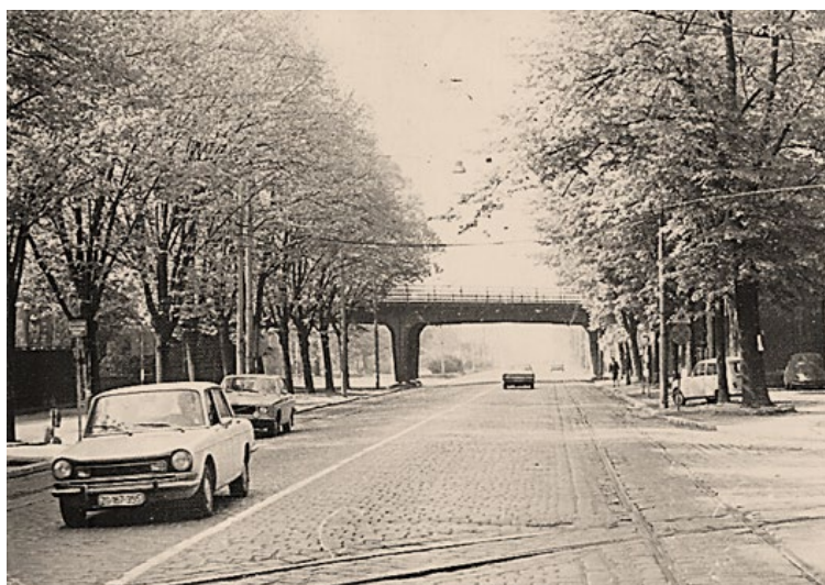
Figure 3. Zagreb's Savska Road and the Railroad Overpass
