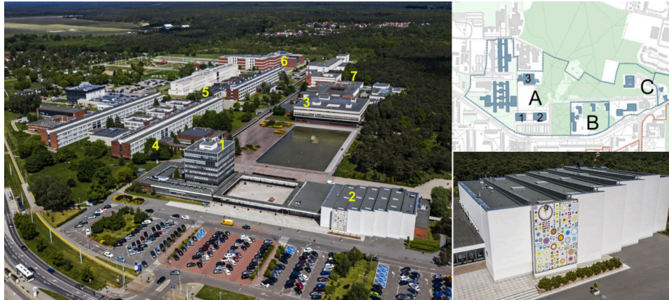
Figure 6. Toruń, NCU campus: a main part (A) with Rectorate (1), Assembly Hall (2), Library (3), Faculties: of Chemistry (4), of Biology and Environmental Protection and of Earth Sciences (5), Colegium Humanisticum (6), of Economic Sciences and Management (7); a residential part – dormitories (B), east – residential part (C) with an academic club, formerly canteen building, a gymnasium and a clinic with a sanatorium (now Institute of Psychology). Bottom right: Assembly Hall (photo. Andrzej Romański https://portal.umk.pl/pl/article/kampus-umk-okiem-urbanisty https://portal.umk.pl/pl/article/ponadczasowy-prezent-dla-kopernika ; plan: https://mapy.zabytek.gov.pl/nid/ , accessed August 28, 2024)
