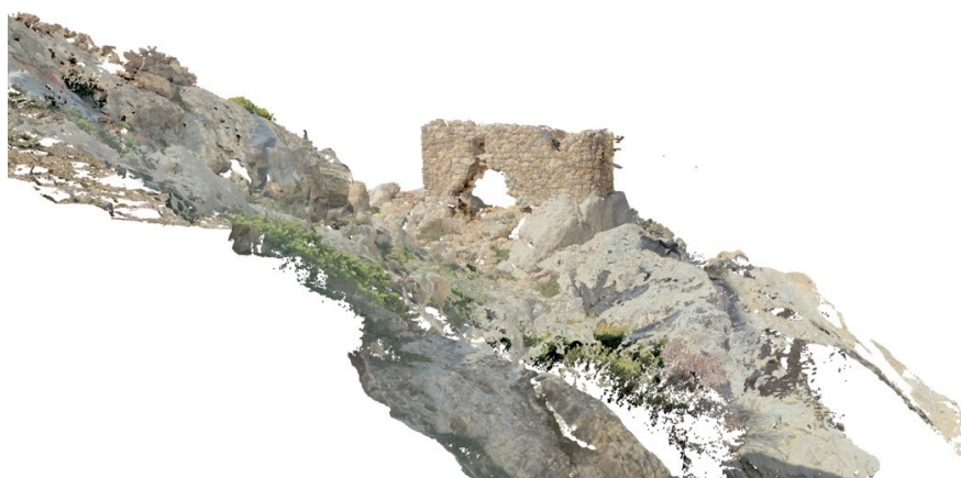
Figure 7. Digital survey. Military structure in Barranco de San Juan, 2024.
