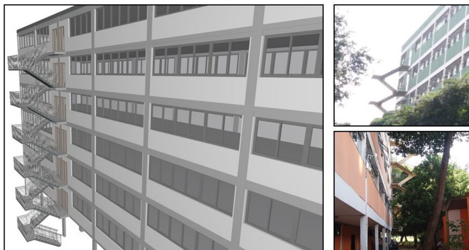
Figure 8. Prefabricated stairs used in the CRUSP by the authors
