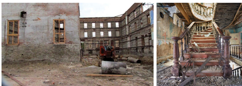
Figure 2. Case Study III_Shelled during the discovery and demolition stage where masonry facades of heritage value are supported, restored and repointed to a more glorious version of itself while the interior stair is deemed structurally compromised and unsalvageable.
