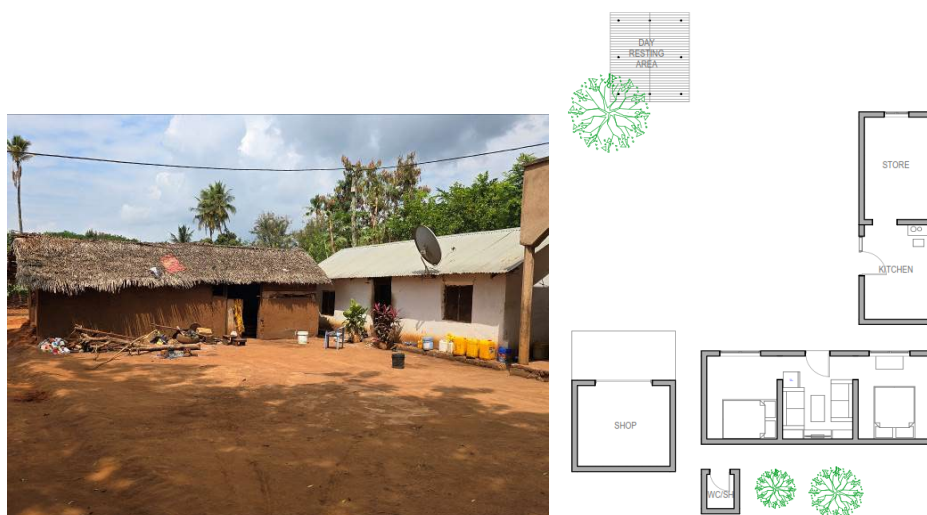
Figure 5. The living/ sleeping unit is made of traditional mud and pole walls with a modern corrugated iron sheet roofing, and concrete flooring, whereas the kitchen is a typical traditional construction. This is a local resident’s homestead located in Kwemazandu village, Korogwe district, Tanga, Tanzania
