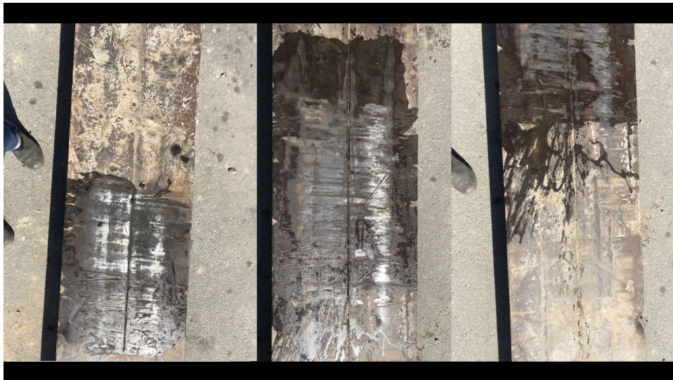
Figure 6. Steel flanges with soap for sliding by Tonia Carless and Robin Serjeant 2023
