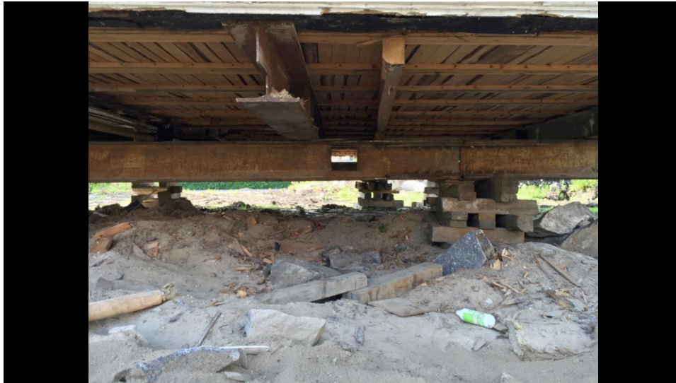
Figure 3. The underside of the house in Umeå, lifted and ready to move, by Tonia Carless, 2021
