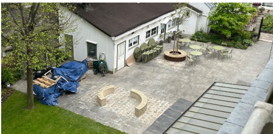
Figure 8. Construction of the base courses is complete, April, 2023. Photo: Barry Bergdoll.
