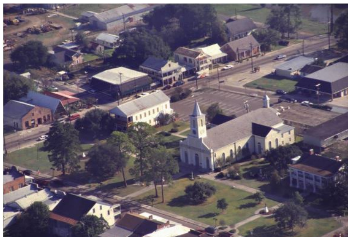
Figure 2. Background buildings defining square with church as dominant set-piece
