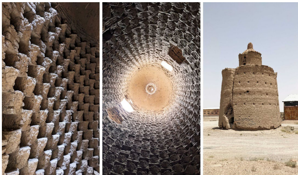
Figure 1. The pattern of solids and voids in the interior of an Iranian pigeon tower resulted from the repetition pigeon nests and perches
