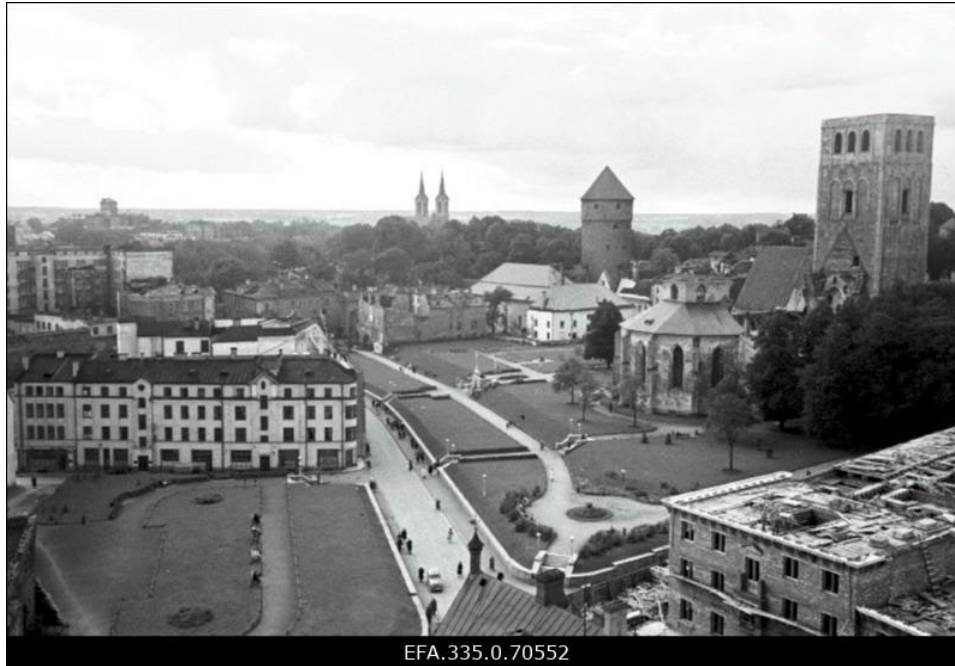
Figure 6. The public green area of Harju Street in 1952. Source: Estonian Film Archive.
