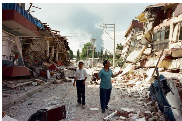
Figure 2. The devastation of the 1999 earthquakes
