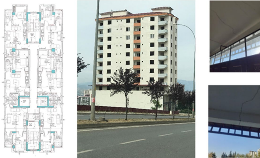
Figure 2. An apartment building with cantilever projections on multiple facades, Kahramanmaraş 2024.
