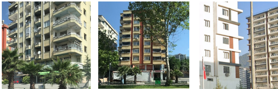
Figure 1. Examples of cantilever projections in reinforced concrete buildings, Kahramanmaraş 2024.
