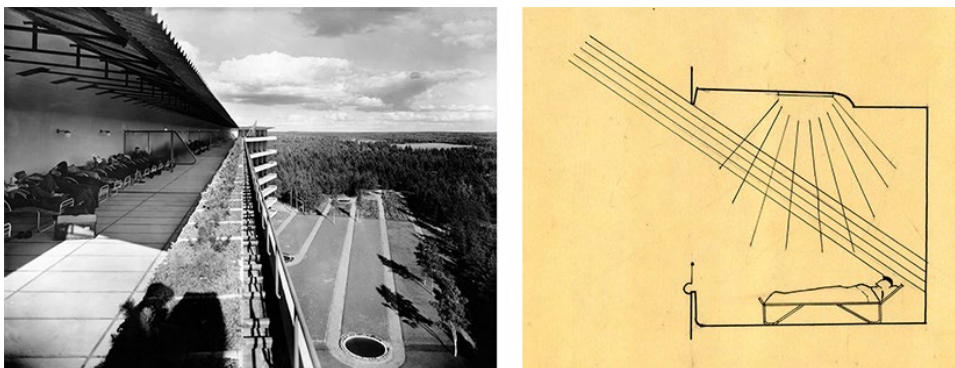
Figure 3. Alto's Finnish sanatorium design principles; maximizing daylight, proximity to nature, and fresh air circulation 17
