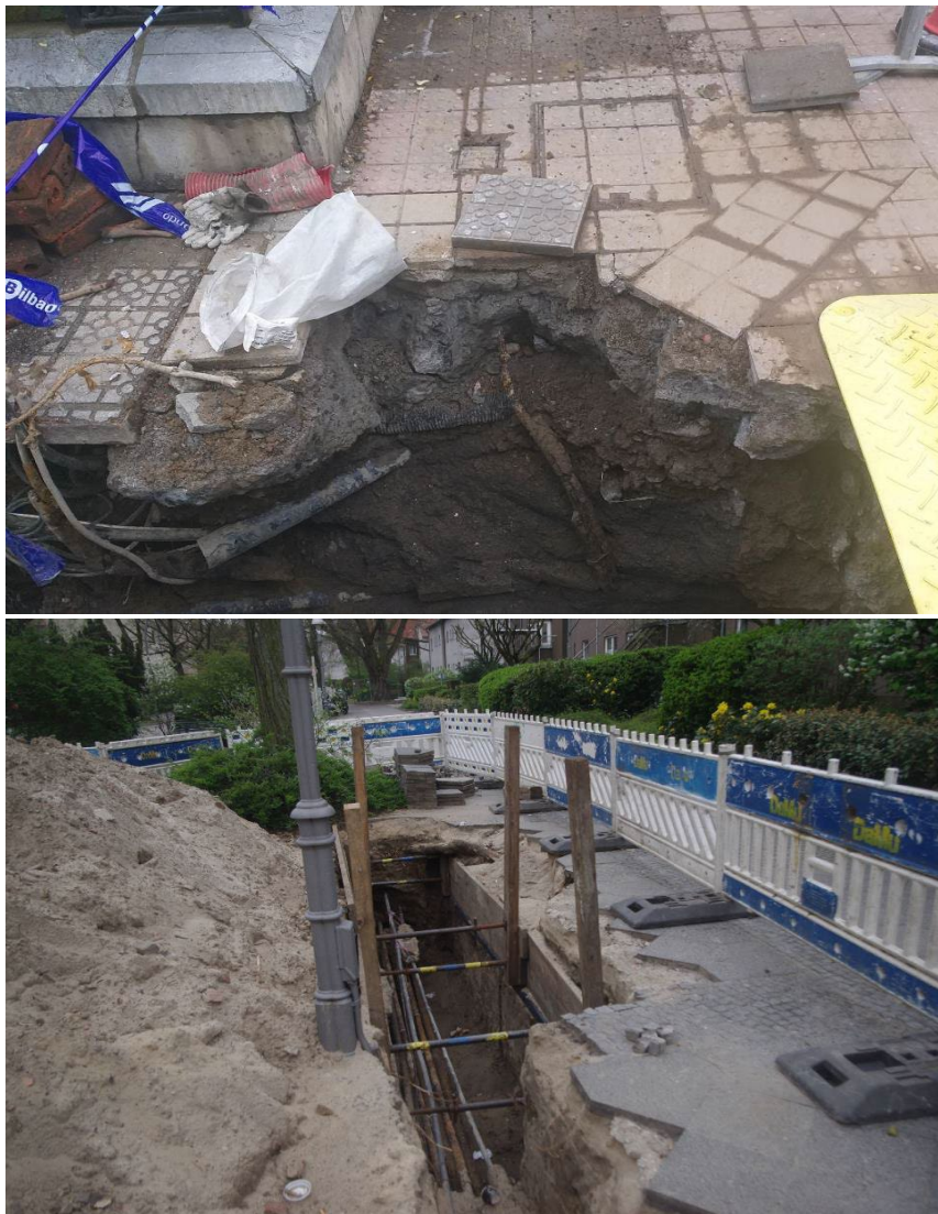
Figures 6 and 7. Comparison between the concrete-based rainproof ground in Bilbao (Spain) and the sand based permeable ground in Berlin (Germany)
