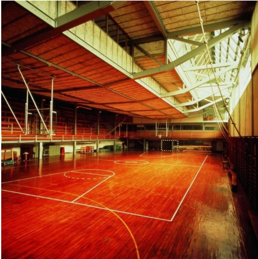
Figure 4. Alejandro de La Sota. Gymnasium in Madrid, 1961. The classrooms are “hanging” in between the trusses, showing coordination between the structure system and the required functions. (Source: Fundación Alejandro de la Sota)
