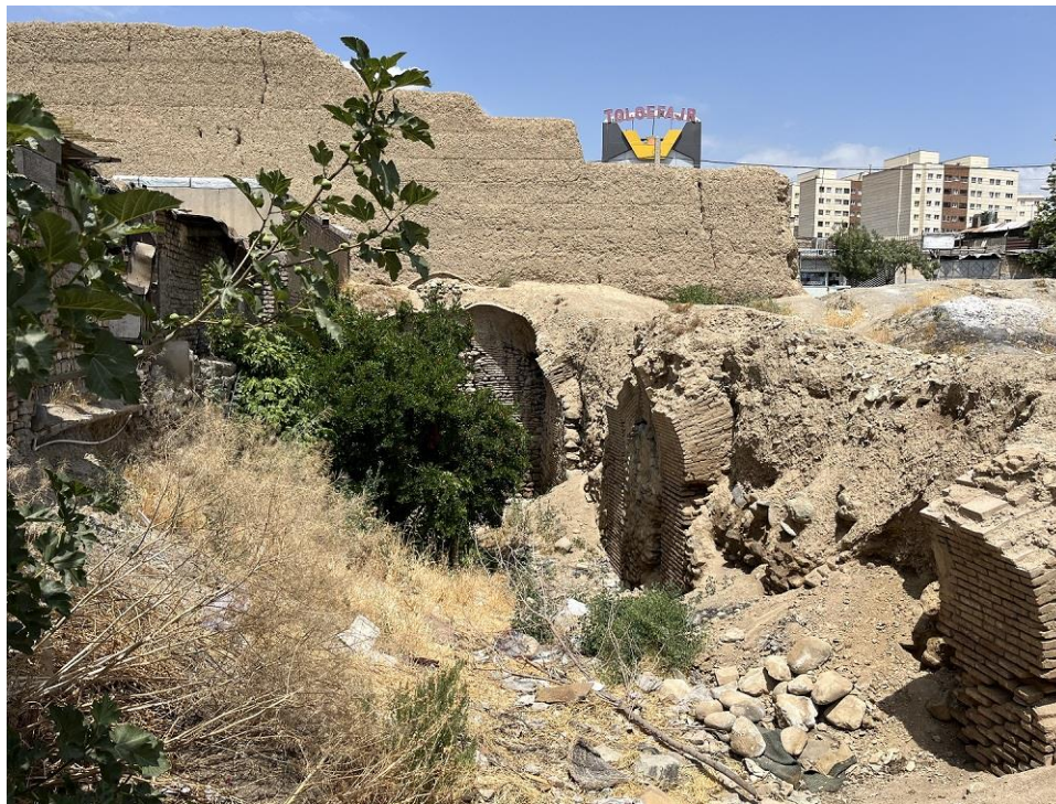
Figure 9. The ice reservoir of the yakhchāl of Kan is seen with the shading wall and its entrance in its new surroundings
