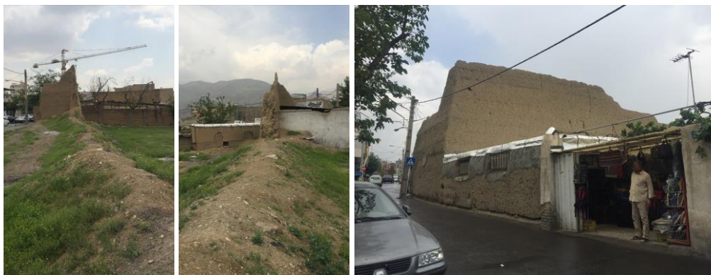
Figure 7. The shading wall of the yakhchāl of Kan
