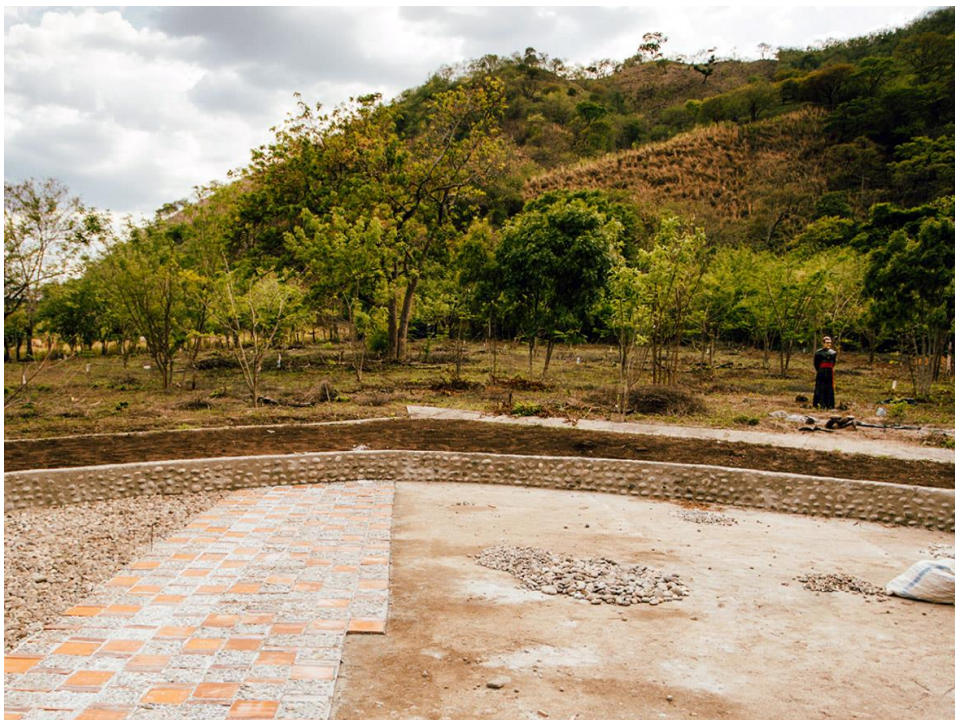
Figure 5. Installation of the memorial and statue of Romero 27
