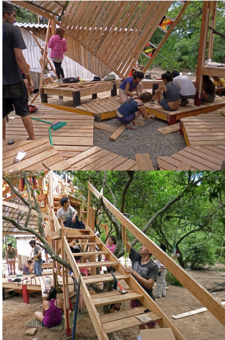
Figure 5. Design and construction of the floor levels and staircase to the treetops, by Oscar Andrade Castro.
