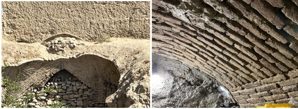
Figure 8. The entrance in the wall to the ice reservoir of the yakhchāl of Kan
