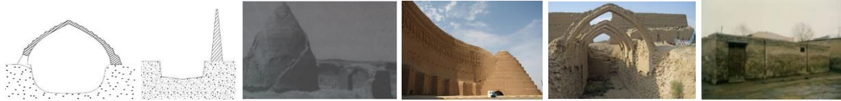
Figure 3. 1. A simple yakhchāl 2. A yakhchāl without a roof 3. A yakhchāl without a shading wall 4. A complete yakhchāl in Maybod 5. Two underground yakhchāls in Qom 6. A tunneled one in Tabriz Hemming Jorgenson, Mokhlessi
