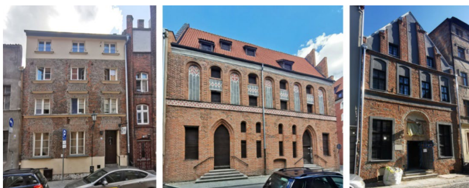
Figure 6. Toruń, tenement houses at 7 Piekary Street, 4 Piekary Street and 12 Franciszkańska Street after (and during) conservation and restoration works (photo. K. Zimna-Kawecka, 2023).
