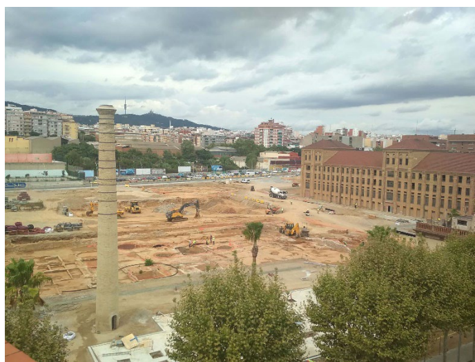
Figure 9. Archeological remains found during excavations.
