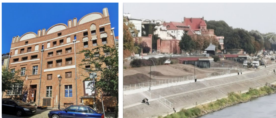
Figure 7. Toruń, tenements at 6 Mostowa Street after works (photo. K. Zimna-Kawecka, 2023). Of the right: construction of pavilions and works on the Vistula waterfront in the zone (fot. K. Zimna-Kawecka, 2023).
