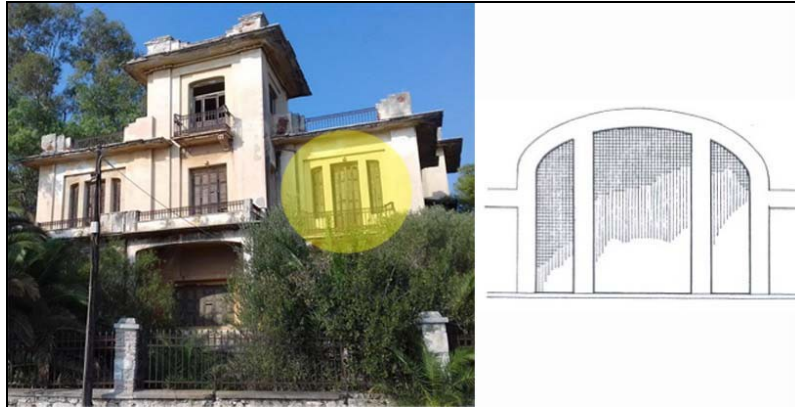
Figure 2. Characteristic forms of openings of the 1920s - The Form of "Canister Handle" (Biris, "Athenian Architecture", 149)
