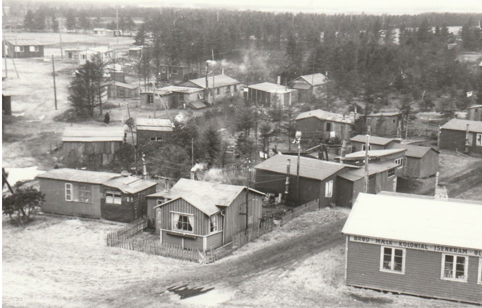
Figure 4. View of Søby circa 1946. Though all buildings differ from each other, there is a strong affinity between them. Photo by the courtesy of Evald Eybye
