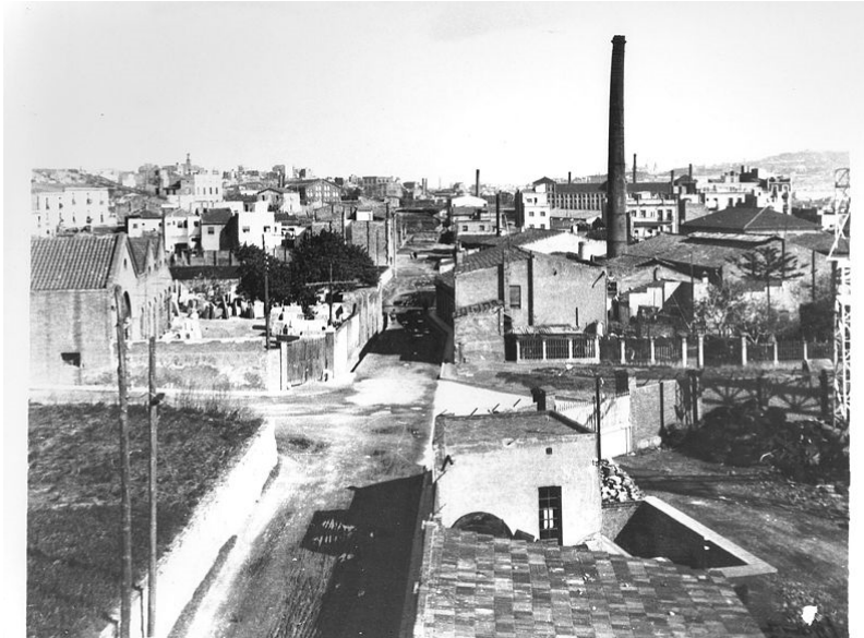
Figure 5. Cosme Toda factory and surrounding, 1955. Source: L'Hospitalet Municipal Archive.
