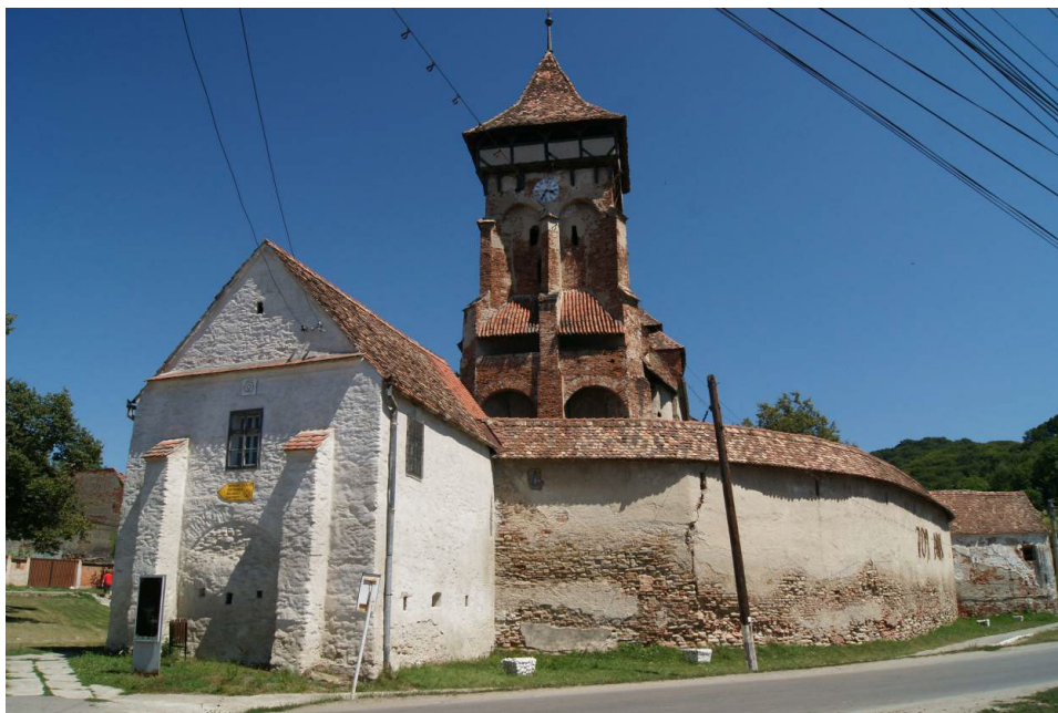
Figure 4. Valea Viilor Fortified church – Exterior photograph with the defensive wall and the church's tower
