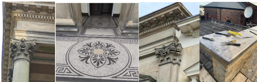
Figure 10. Repairs and Restoration (left to right): Portico 2005-9, Church Roof 2014-5, Presbytery Roof 2022, by author.
