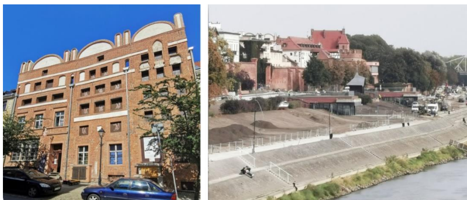
Figure 7. Toruń, tenements at 6 Mostowa Street after works (photo. K. Zimna-Kawecka, 2023). Of the right: construction of pavilions and works on the Vistula waterfront in the zone (fot. K. Zimna-Kawecka, 2023).
