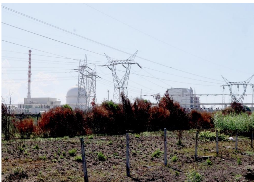
Figure 1. Ex-Nuclear Power Plant, Borgo Sabotino, Latina 2022. Ph. F. Fava
