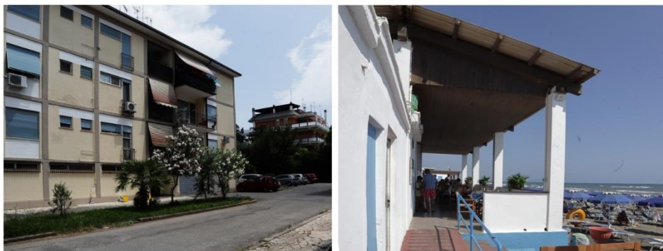
Figure 4. ENI housing and beach facilities, Ph. F. Fava. June 2023
