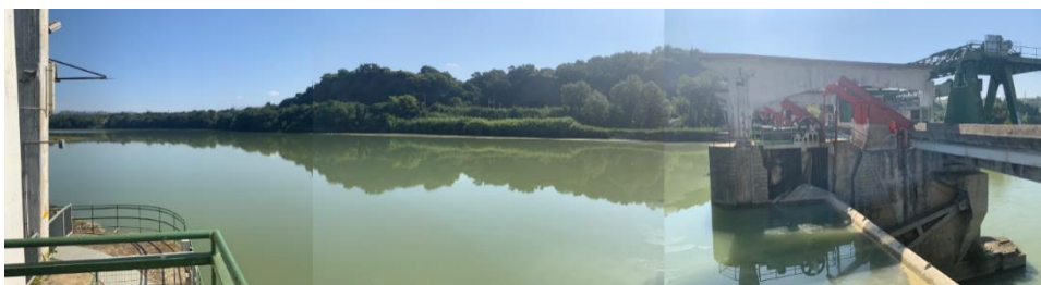
Figure 7. Tiber basin and the dam lake. Ph. G. Caudo (August 2023)
