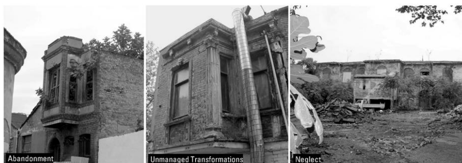
Figure 6. Photos taken during on-site survey by Ekin Olcay 2020
