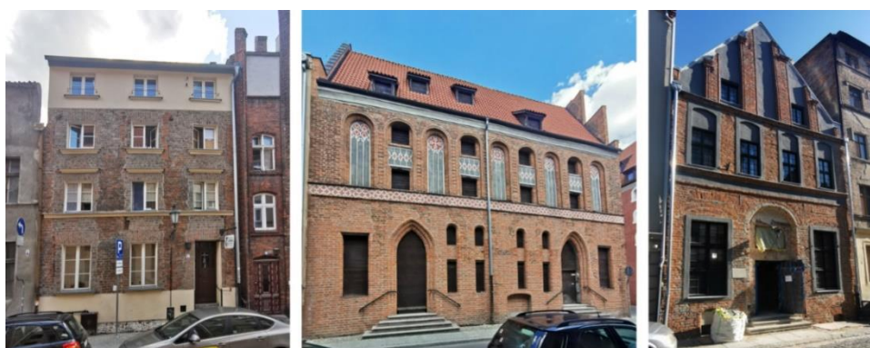
Figure 6. Toruń, tenement houses at 7 Piekary Street, 4 Piekary Street and 12 Franciszkańska Street after (and during) conservation and restoration works (photo. K. Zimna-Kawecka, 2023).
