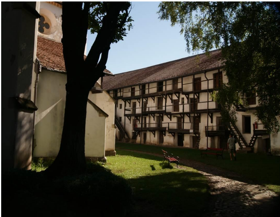
Figure 2. Prejmer Fortified church – The interior view of the defensive wall with the pantry rooms
