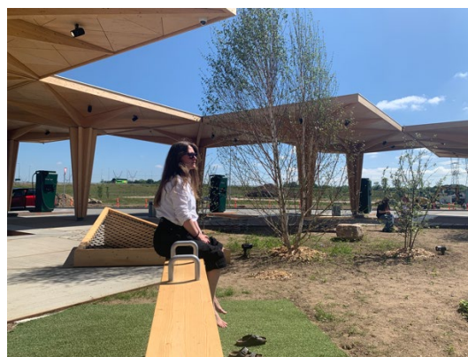
Figure 2. The recharging station for electrical vehicles with the wooden canopies and the recreative landscape elements in Odense, DK.
