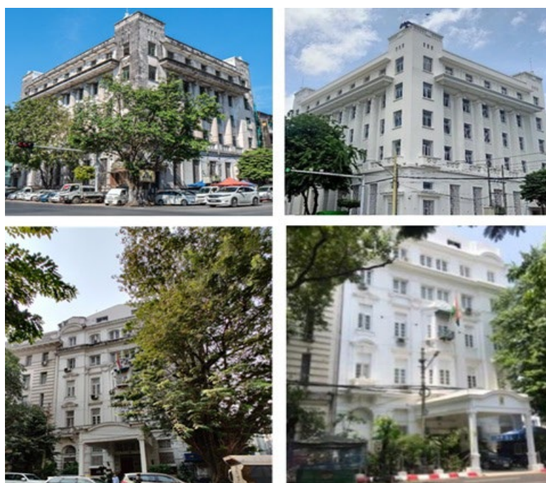
Figure 8. Rehabilitated Historic Building on Merchant Street Yangon (Before and After)
