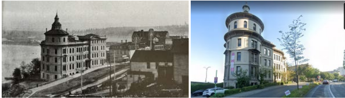
Figure 2. The Northern Pacific Headquarters Building.
