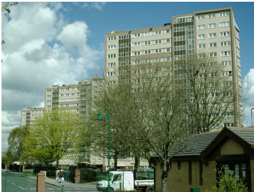
Figure 1. Medway, and Thames Towers on the Cromwell Street Estate, Nechells Green Severn,
