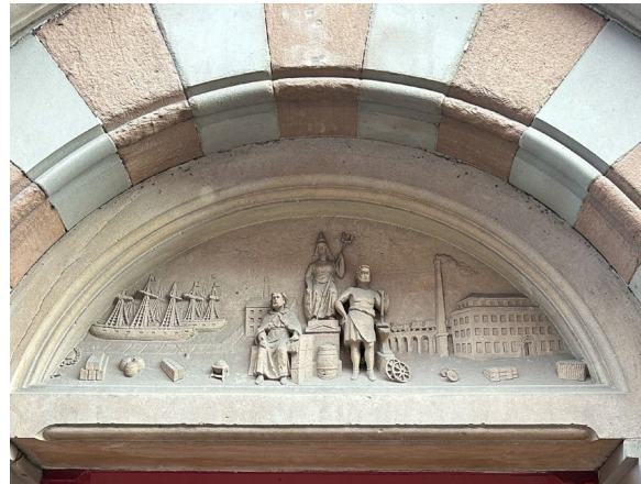
Figure 2. Tympanium at the Adam's Building, Nottingham Lace Warehouse Photo: Briggs-Goode
