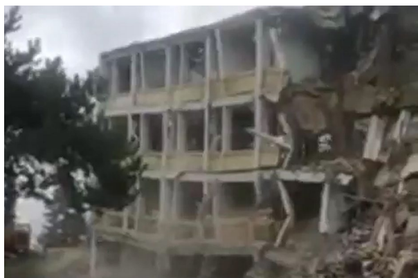
Figure 50. The demolition moment of the Ballıdağ sanatorium building captured from a video Source: Kastamonu Açık Söz newspaper, 6 September 2021
