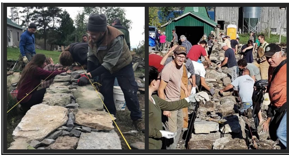
Figure 7: Building the wall together
