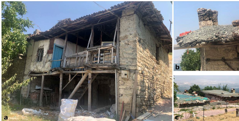
Figure 9. a. The houses at the skirt of Honaz Castle, 2020, b. Detail of a terrace roof remain with earth covering, 2020, c. Terrace roofs at the skirt of Honaz Castle 2020
