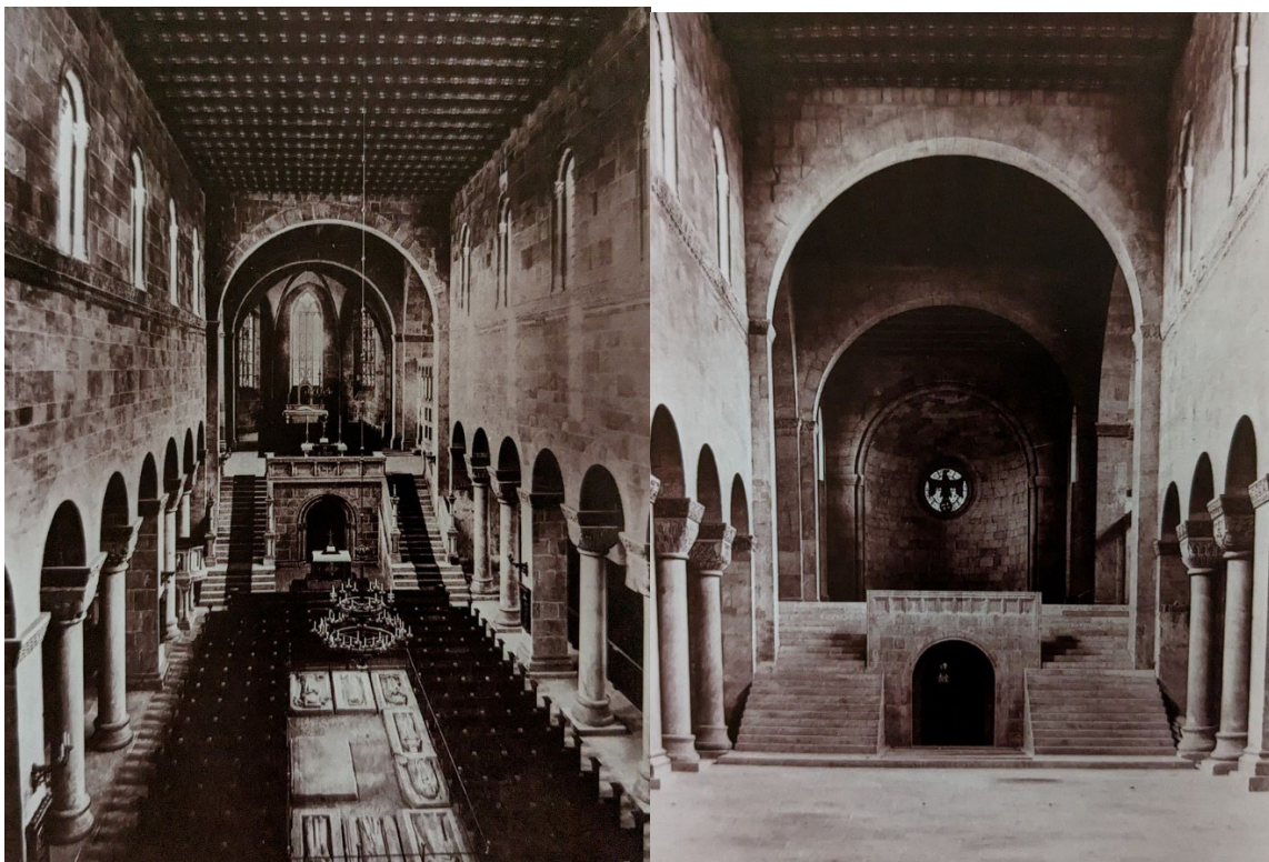
Figure 5. The St. Servatius church before and after the structural changes of the 1930s.
