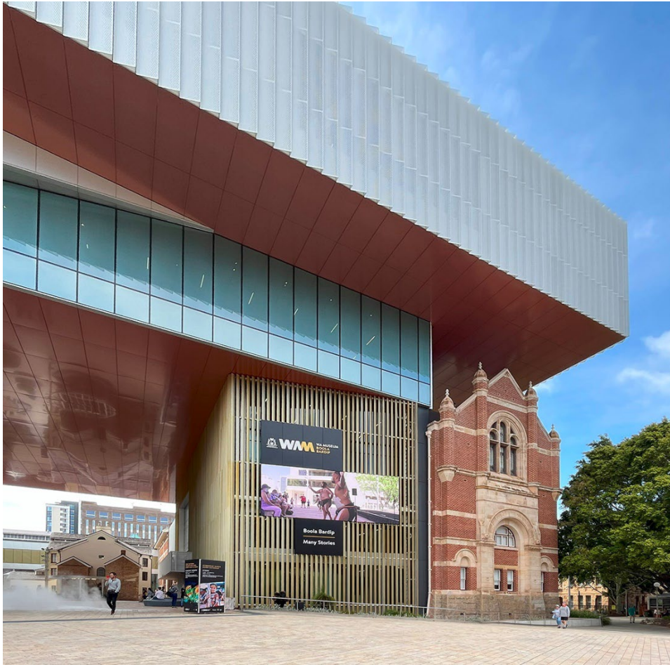
Figure 3. New galleries cantilevering over Hackett Hall (right) at Western Australian Museum Boola Bardip by Hassell + OMA (2020). Photo by Susan Holden, 2022
