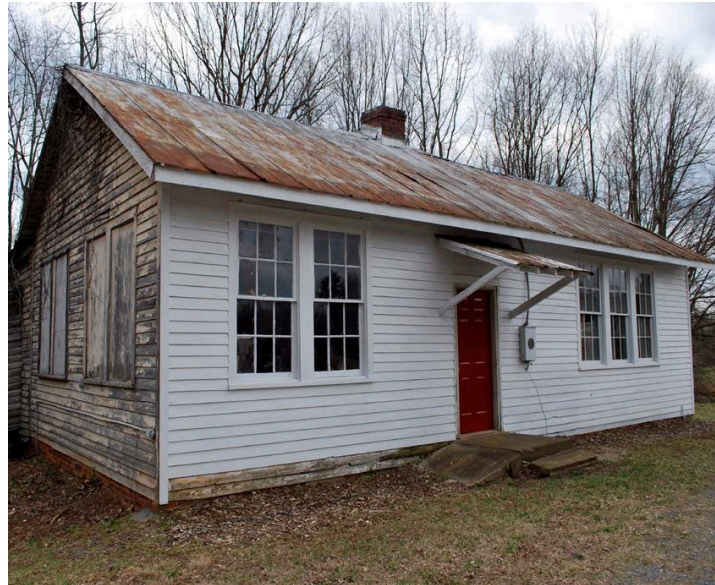
Figure 1. Exterior view Dillwyn Training School Shop Building (before).
