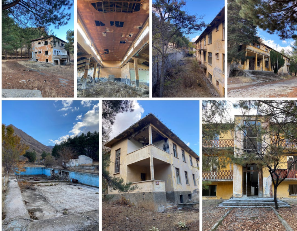
Figure 6. Current condition of the settlement
