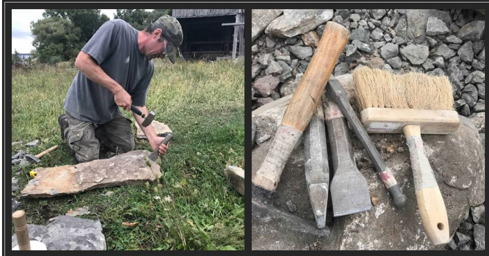
Figure 1. Tools used in dry-stone construction
