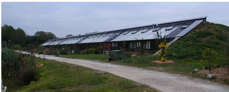
Figure 4. Hockerton Housing Scheme UK showing earth berming (source: Authors).
