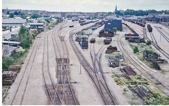
Figure 1. The freight train area when it was still in function in the year 1976. Copyright Aarhus Kommune.
