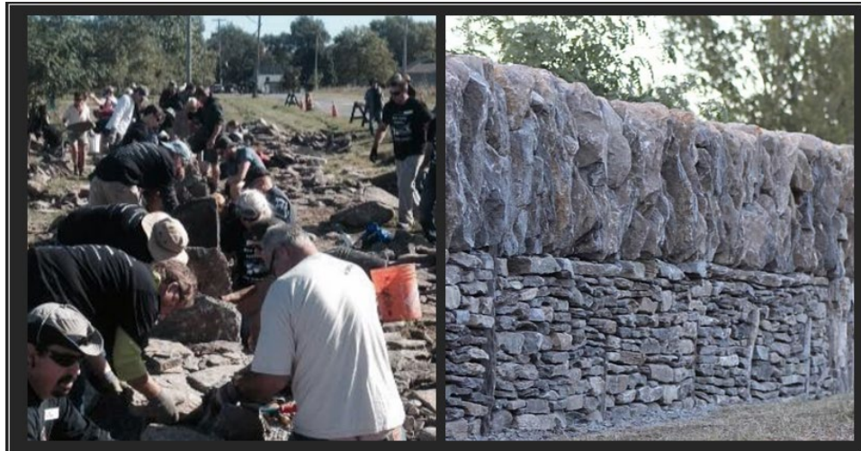
Figure 2. The start and completion of the sample wall
