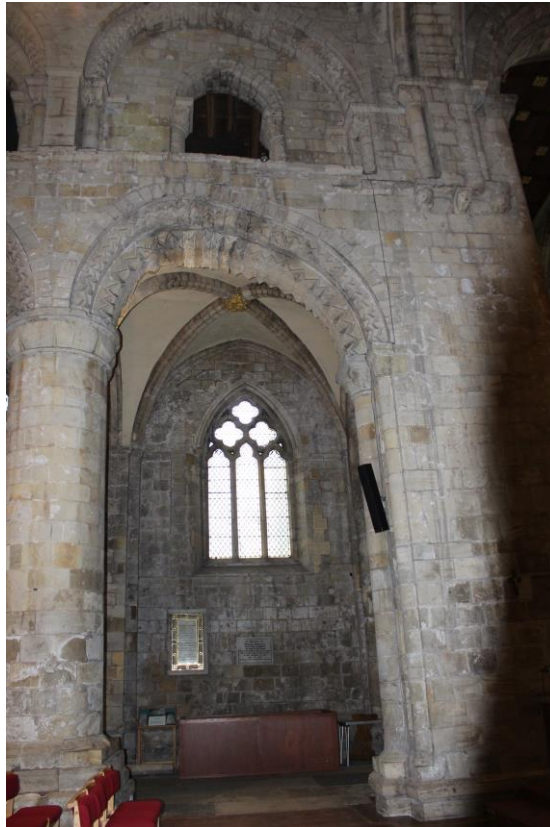
Figure 7. Visible deformation at Selby Abbey
