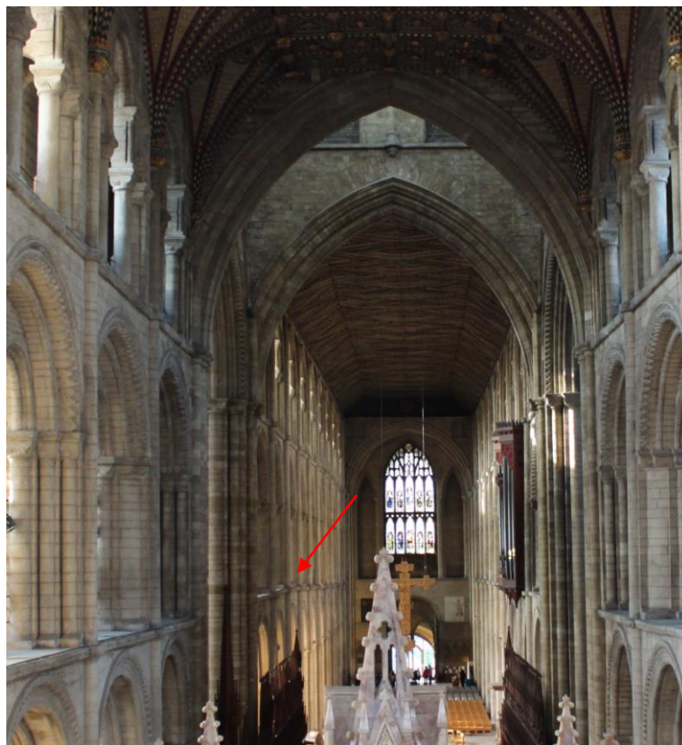
Figure 8. Nave-Tower deformation at Peterborough Cathedral
