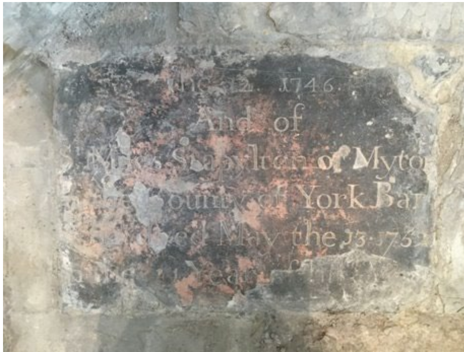
Figure 1. Example of ledger stone, with signs of delamination, by David Littlefield
