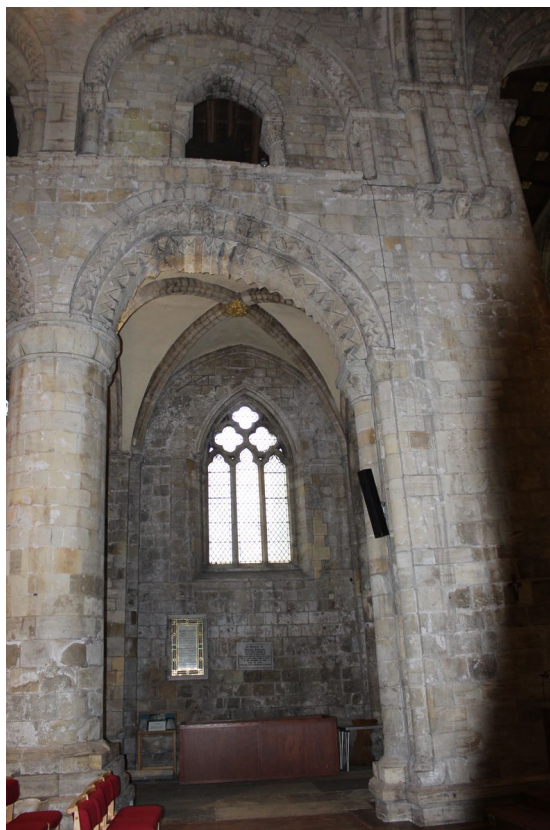
Figure 7. Visible deformation at Selby Abbey
