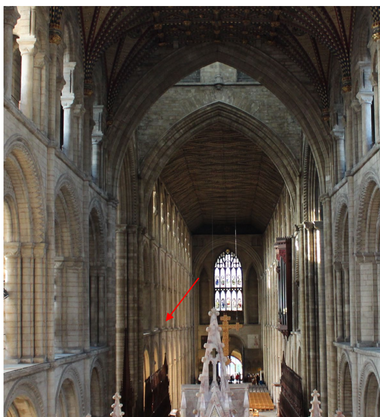
Figure 8. Nave-Tower deformation at Peterborough Cathedral
