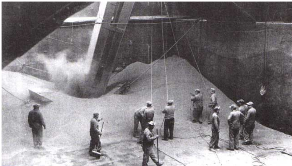
Figure 8. Scoopers in the hull of a grain ship assist the marine leg.
