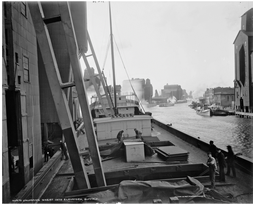
Figure 4. Marine leg unloading grain
