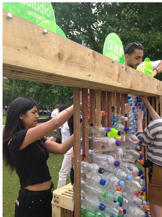
Figure 8. Students inserting bottles in frame
