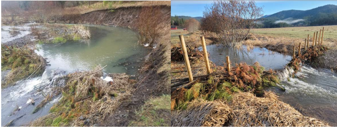
Figure 18. Beaver Dam Analogues in Washington State
