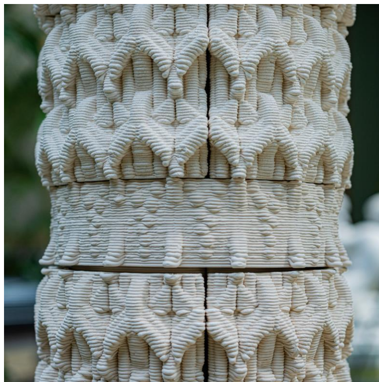
Figure 7. Conspicuous joints between column elements designed to allude to its inner structure
