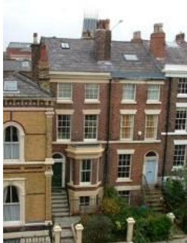
Figure 6: Hope Place, Liverpool Grade II listed terrace
