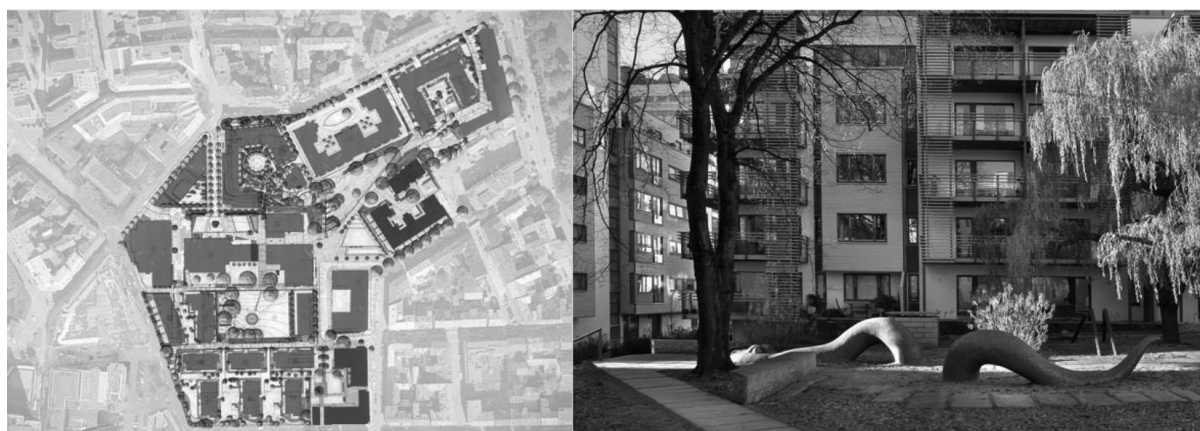
Figure 5 The Pilestredet Park housing project as an example of innercity transformation.
