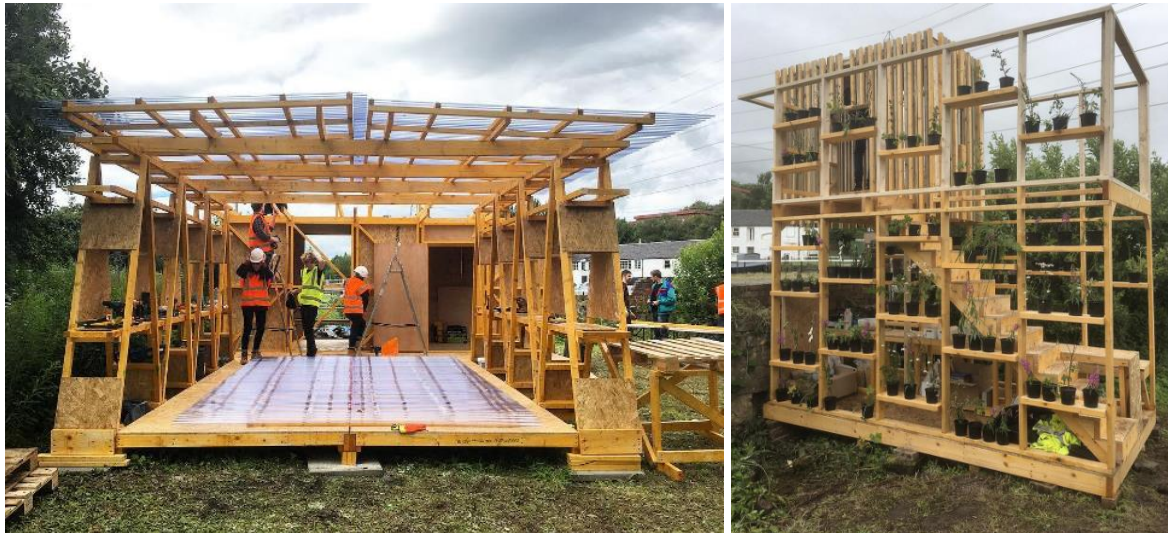
Figure 2: Test Unit, showing main pavilion under construction (left) and 'The Nettle Inn' (right).
