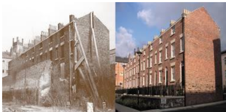
Figure 5: Before and after – Dukes Terrace, Duke Street, Liverpool
