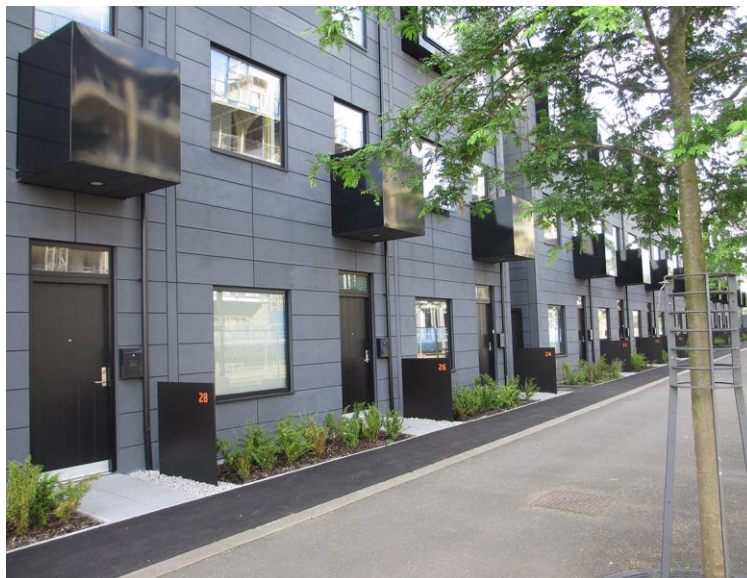
Figure 4. Setting the terrace back from the public realm, and the inclusion of planting, screens and projecting balconies over the entrance, reinforces the sense of threshold for ShedKM's hoUSes.
