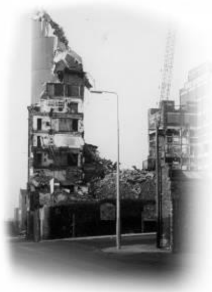
Figure 10: The demolition of Tate and Lyle, Liverpool
