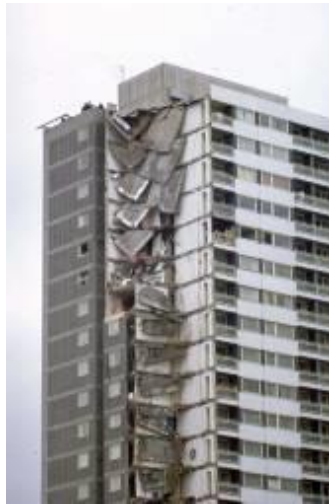
Figure 9: Ronan Point gas explosion
