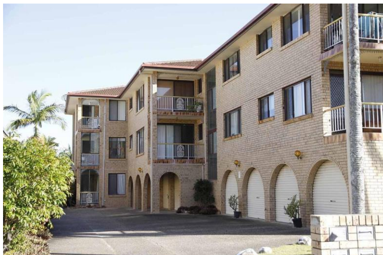
Figure 6. A Gold Coast Residential Unit Block. Photo credit to William Hickman
