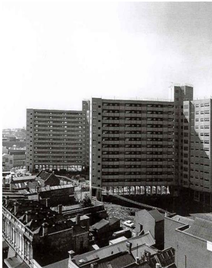
Figure 1. Y-Blocks, Horace Petty Estate, Prahran (Late 1960s) (Source: Stonnington History Centre [no registration number])
