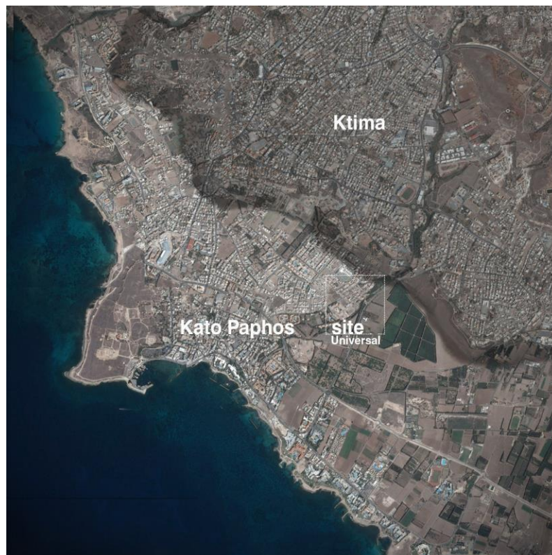
Figure 1. Aerial view of Paphos that highlights the geological rim that separates the old part of the city from its Port and Kato Paphos.
