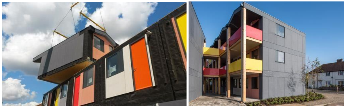
Figure 1. Prefabricated housing project for homeless people in south London by Rogers Stirk Harbour + Partners.
