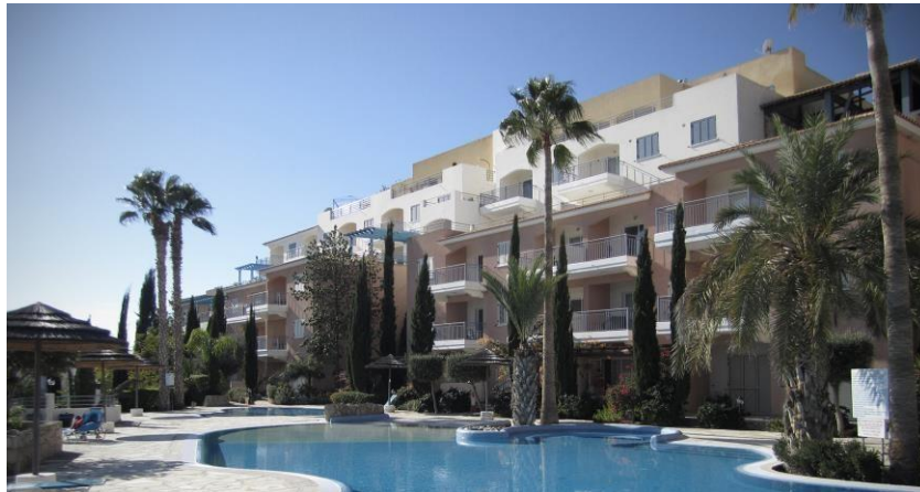
Figure 3. Typical communal facilities to support the lifestyle of summer dwellers and their ephemeral stay in the housing complex.
