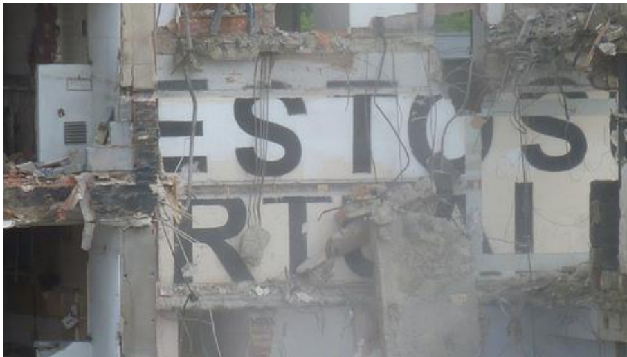
Figure 5. Detail of 'Embodied Text' during demolition
