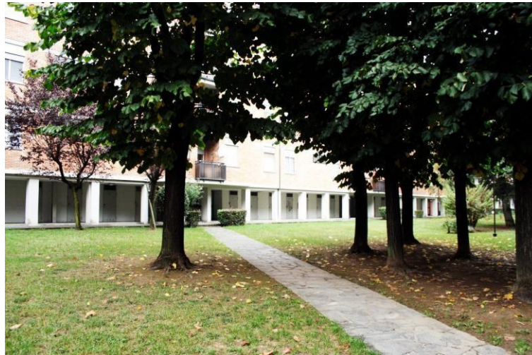
Figure 4. Access to the individual buildings is through the inner gardens
