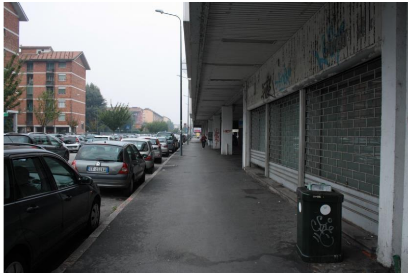
Figure 1. Public space is disregarded, windows are closed and the street is invaded by parked cars
