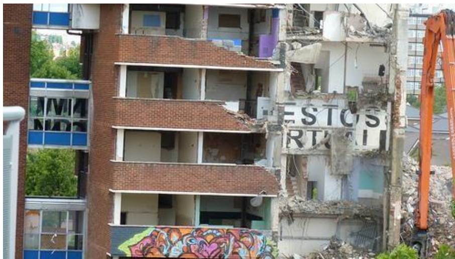
Figure 4. Demolition of The Market Estate revealing 'Embodied Text'
