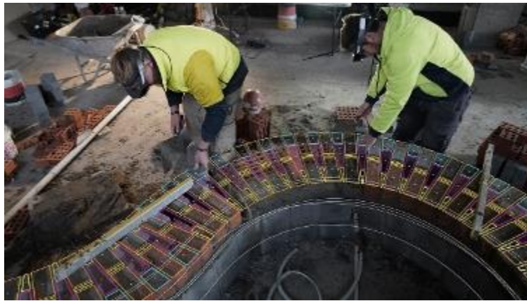
Figure 1. Holographic Construction of the Hobart Hospital by Fologram. (left)
