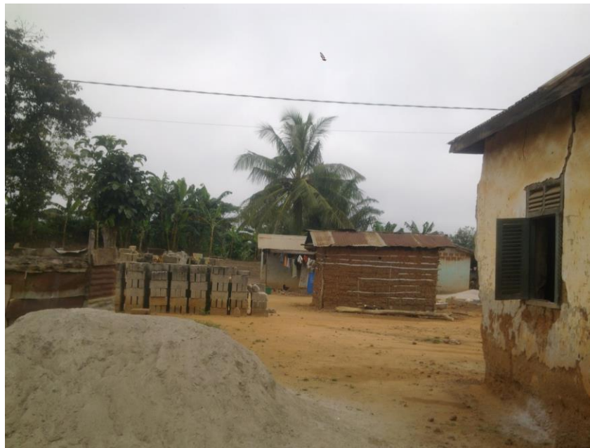
Fig 5. A pile of cast concrete blocks typically stored next to old earth houses, which are left without repairing or re-plastering so they naturally deteriorate and collapse. The owners will build their new home in their place made from concrete blocks.
