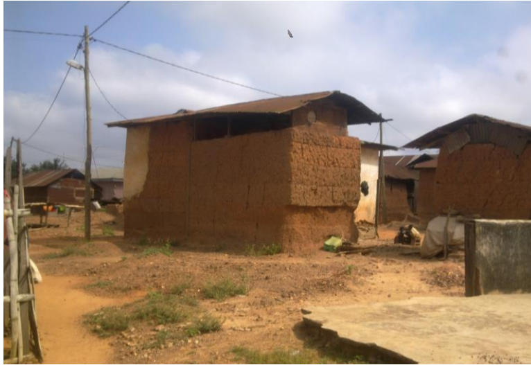
Fig 4. An atakpame earth building gradually falling in ruins due to lack of maintenance, intense rainfalls and lack of foundations causing the lower part of the walls to deteriorate faster
