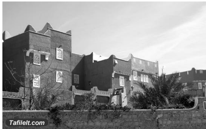
Figure 4. The use of thick walls for cooling (source: Tafilelt.com)
